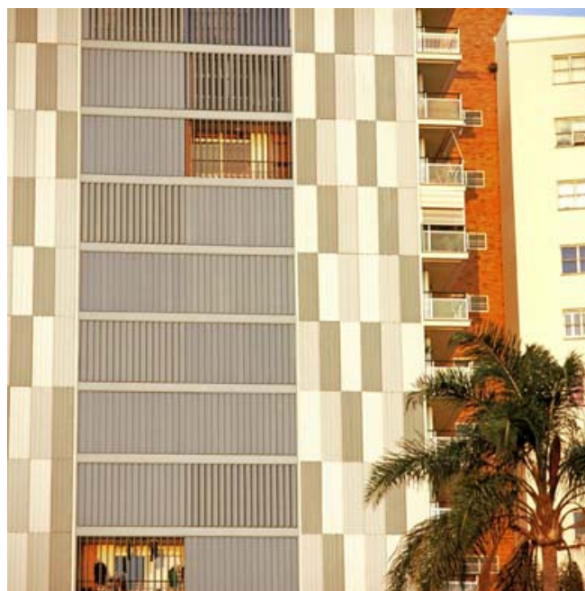
Apartment building in Australia with high thermal mass construction and controllable external solar blinds.
