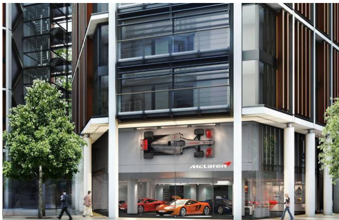
Use of external shading to reduce solar gains on a residential apartment
